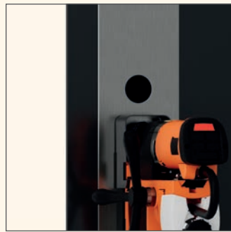
2. Drill a new hole if necessary
